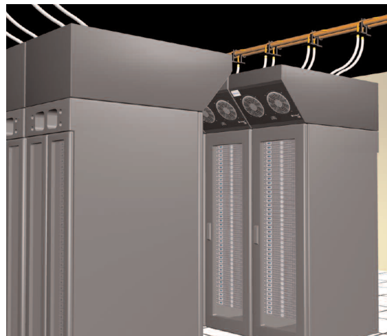
Figure 14. Supplemental cooling enables higher rack densities and improved cooling efficiency.
