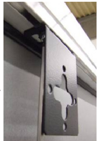
L-shaped Bracket on Horizontal Frame Member
